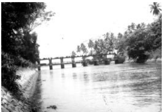
Fig. 8: The regulator without shutters enabling free flow of water in both directions: towards sea and towards estuary.
