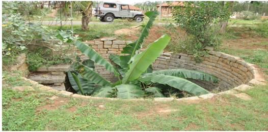
Fig. 7: Dried up and abandoned dug well at Malur village.
